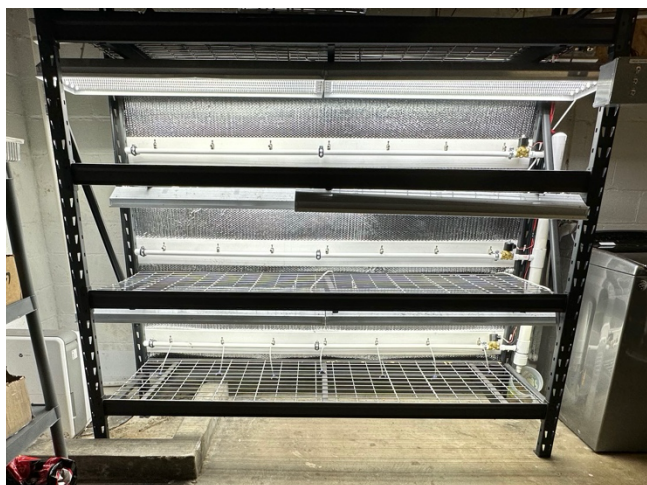
Figure 4: Each shelf in the VF is equipped with white LED lights that are lit for twelve hours each day.
